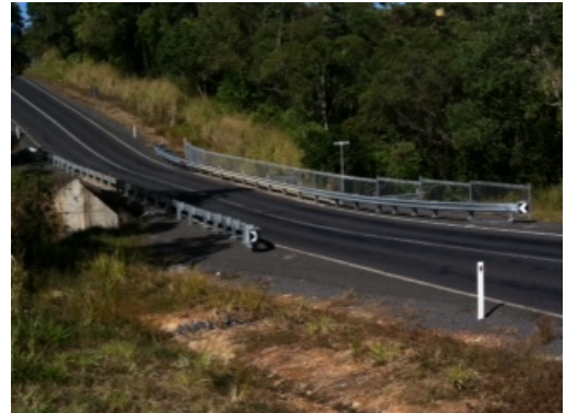
The new Owens Creek Bridge on Myola Road, Kuranda
