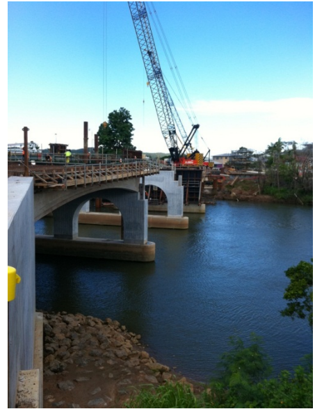
Jubilee Bridge under construction, Innisfail
